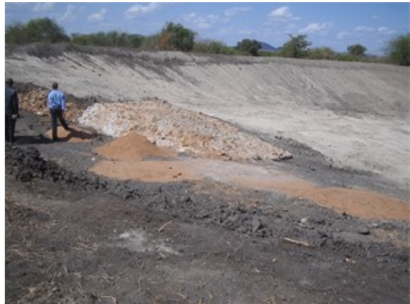
The dam before the rain
