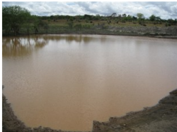
The dam after the rain
